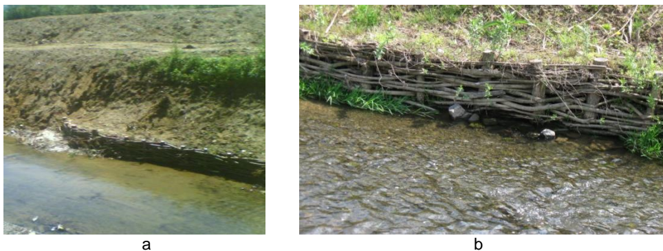
Fig. 1 Biological works in shore defence on Brețcu River, place. Tg. Secuiesc: a - braids/wattle; b - details on the location of biological protection (Luca, 2011)
