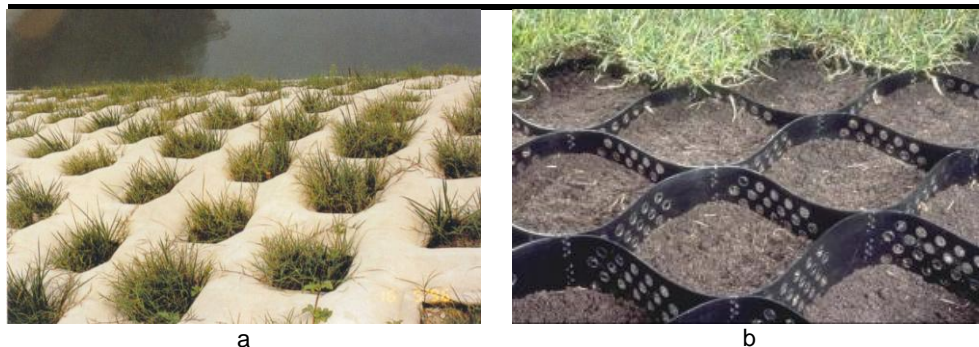
Fig. 4 Mixed riverside protections: a - grilled and sown geo-bags; b - geocells filled with grass roots.
