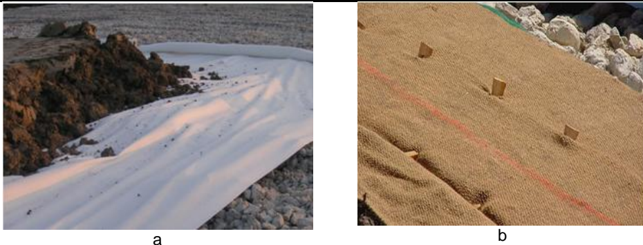
Fig. 3 Biodegradable geotextiles: a - material layout and leaching on the slope; b - tiling of a woollen cloth geotextile (Sion, 2019).
